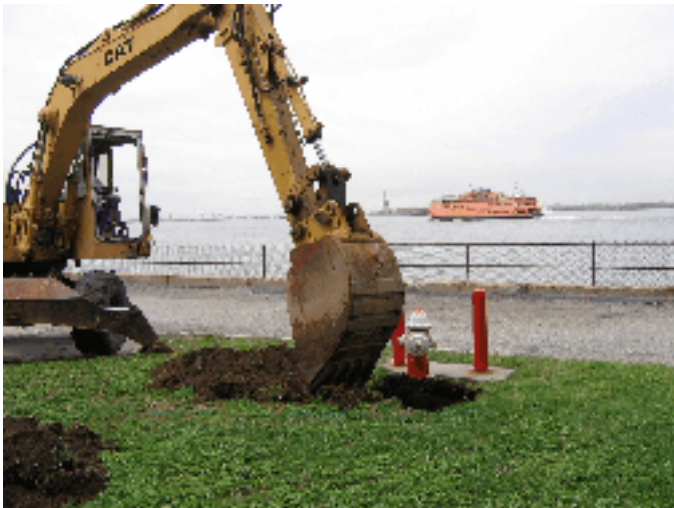
Monitoring excavations on the west side
